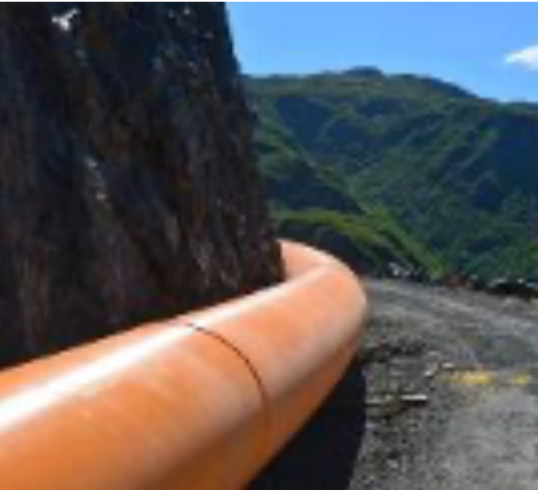
Our BorSafe™ PE material was used to produce a first-of-its-kind 1,600 mm diameter PE pipe for a hydroelectric power project in Alaska
